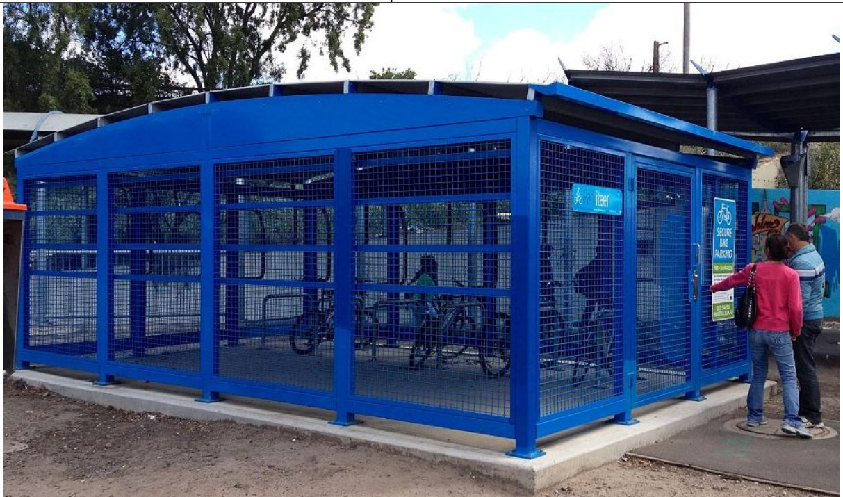
Figure 8 Cycle Parking – Cycle Compound
